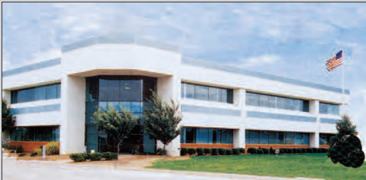
Global Headquarters, Hauppauge, NY USA 100,000-square-foot facility, including design, manufacturing and corporate management.
