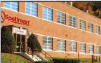
Valhalla, NY USA 35,000-square-foot facility dedicated to design, manufacturing, sales and service.
